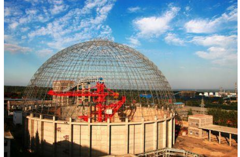
Steel structure dome
