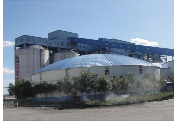
Steel structure dome
