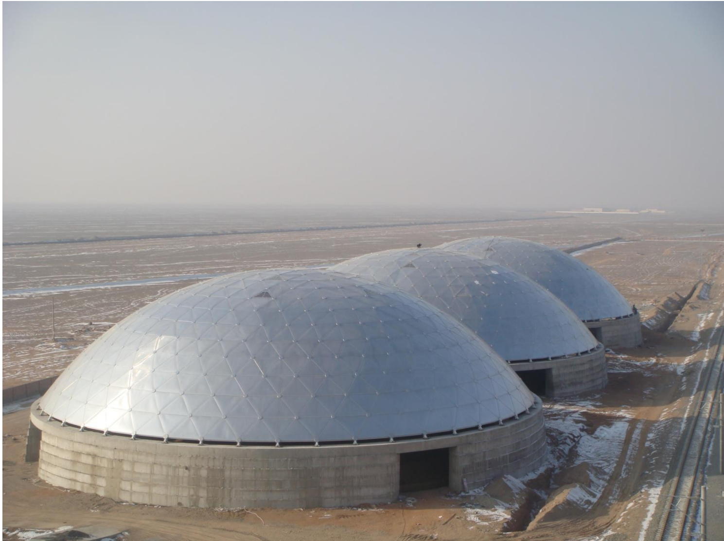
Three 60-meter-diameter all-aluminum domes
