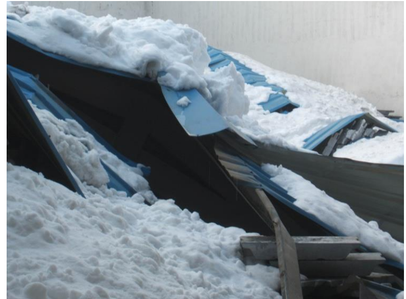
Steel structure dome
