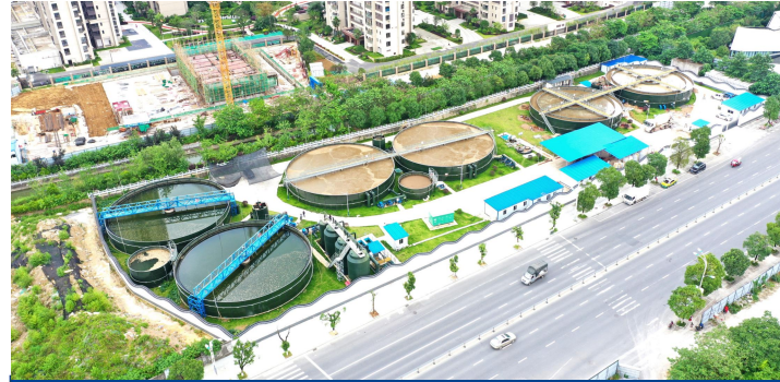
Guangxi sewage project
