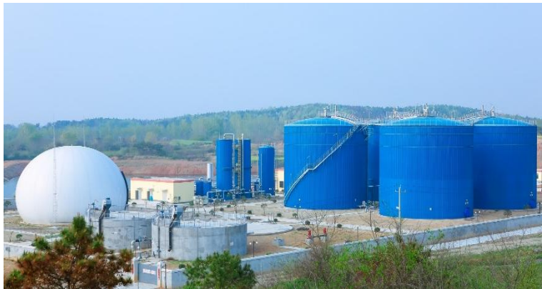
COFCO Wuhan Guangshui pig manure project
