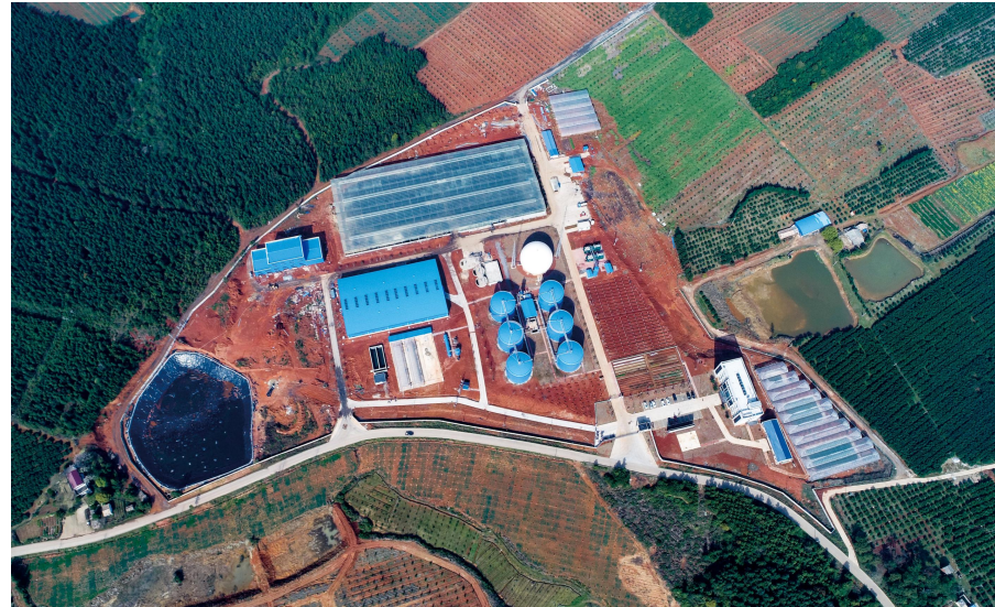
Xinyu centralized manure treatment plant
