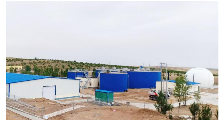
COFCO Chifeng pig farm project
