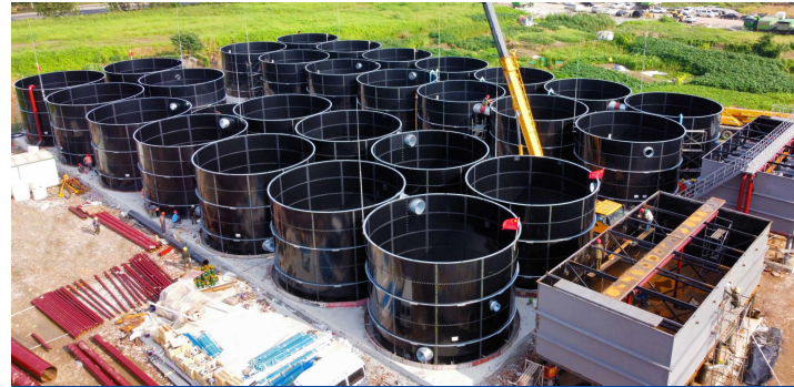
Jiangsu sewage project
