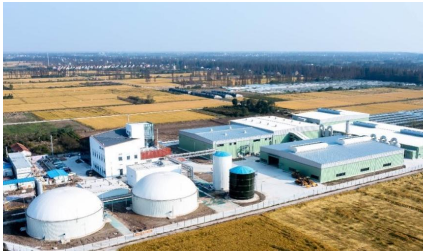
Shanghai Electric Group biogas project Location: Chongming Island, Shanghai
