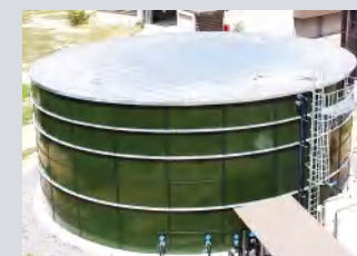
Trough Deck Roof
