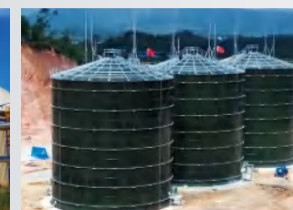
Tapered Steel Roof
