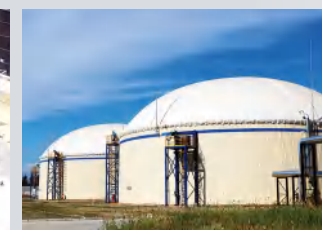
Double Membrane Roof
