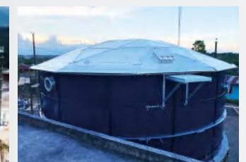
Geodesic Dome Roof
